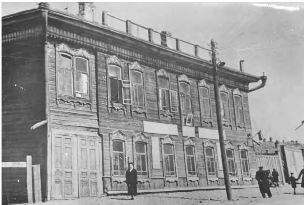
TB Center, 24 Nechayevskaya St., Tomsk, 1920s
